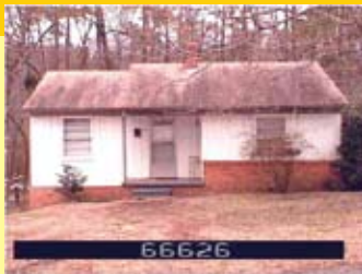
In 2010, this Long Acres home was condemned and torn down. ▲
