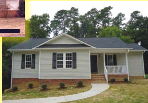
◀ This is the same lot in September 2011 after a new, energy efficient home was built in partnership with Barbara G., a Triangle Transit bus driver and mother of two girls. Barbara is an enthusiastic new homeowner eager to participate in the Community Coalition.
