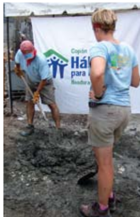
▲ Mixing cement in Santa Rosa
